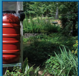
Rain barrels collect roof runoff
